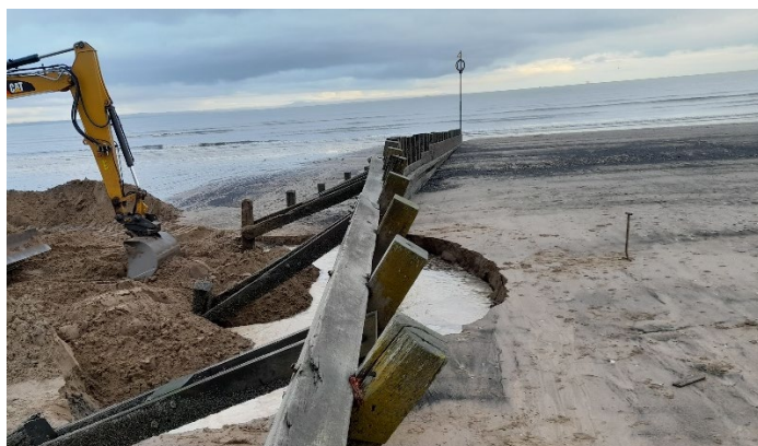
Figure 3 - Exploratory works to damaged Portobello Groyne No. 4 following Storm Arwen
